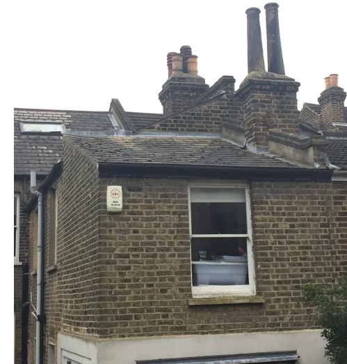
Photo of roof to clarify existing configuration
